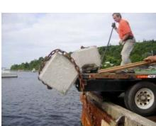
They will only charge you about 25 dollars for this. You should bring them the bottom chain to cast into the block. After it is poured and cured you will have to arrange for a truck to pick it up. The concrete company will load it for you. It is best if this is on a flat bed truck to have it near the back and
